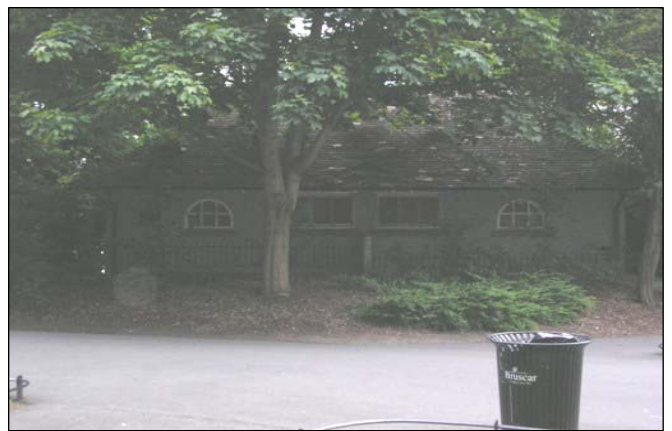
Plate 26: Public toilet block on St. Stephen's Green West
