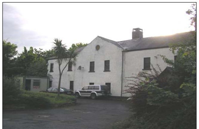
Plate 16: Santry Lodge on the Old Ballymun Road in Santry
