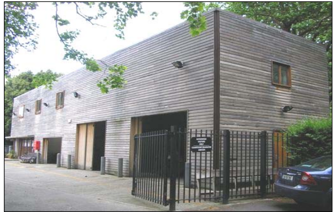
Plate 22: Maintenance offices and workshops at southern side of Green
